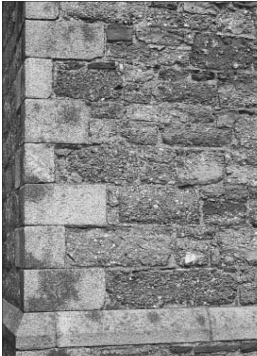
Conglomerate red sandstone with granite quoins, County Wexford.
